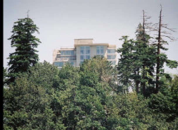
Photo of the rear tower at same location (June 2005)
